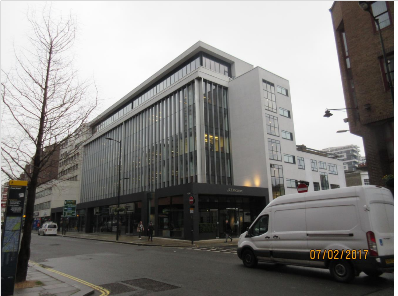
Above: Post implementation of 2011 planning permission.
