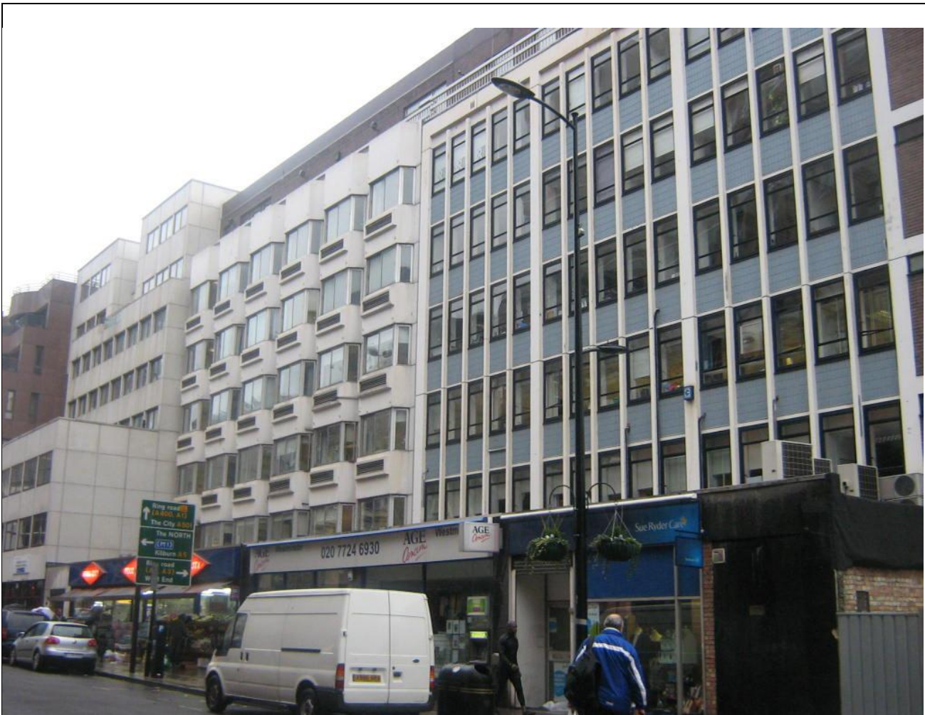
Above: Pre implementation of 2011 planning permission.
